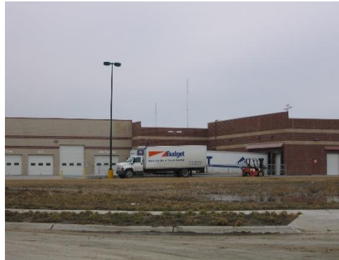
A loading area hidden from the primary view of the store
