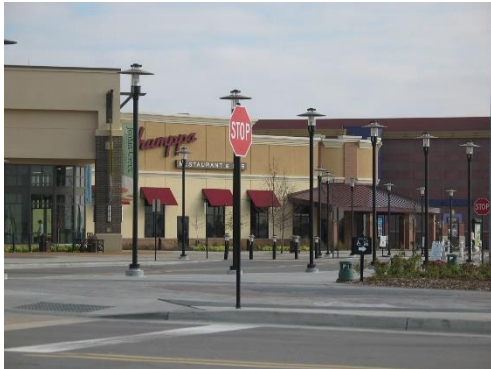
The lighting above is taller but is still of a human scale
