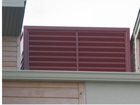
Closer view of the screening shown at the left
