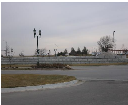
The retaining wall provides for physical and visual separation of the parking area and circulation system
