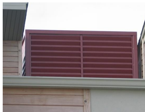
Closer view of the screening shown at the left
