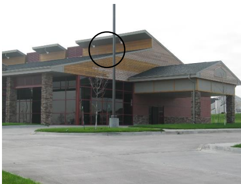
An example of screening an air handling unit
