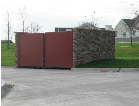
An example of screening trash dumpster areas
