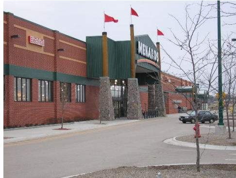
An example of a wall sign and an incidental sign (to the left)
