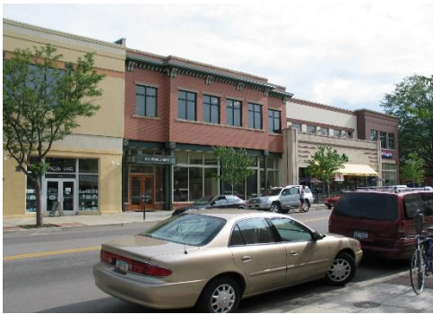
The brick building in the center is an example of an infill project.
