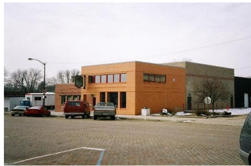
Another example of an infill using appropriate materials.
