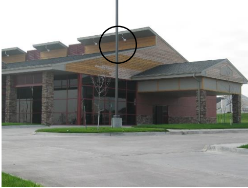
An example of screening an air handling unit
