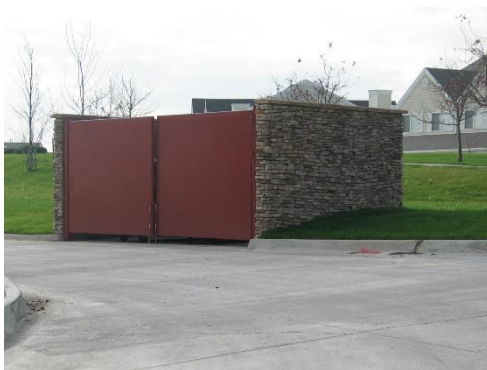
An example of screening trash dumpster areas
